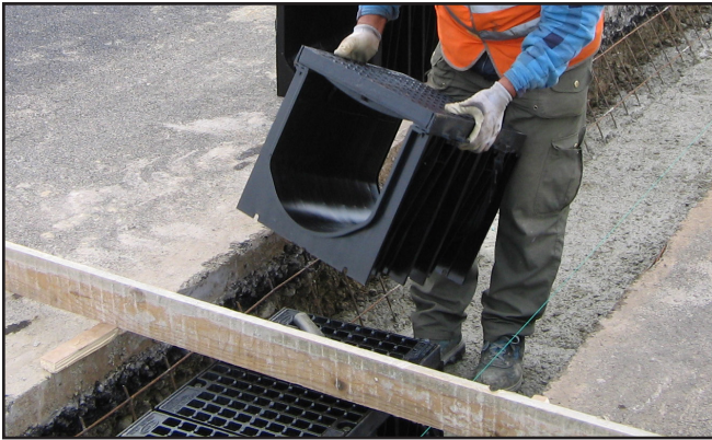
Lightweight, one-meter channel sections are relatively easy to handle, move, and set in place. Ductile iron frame/grate makes the system suitable for heavy-duty applications.
